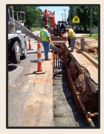
Joint-use duct bank installation on the N. Main St. Widening Project.
