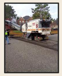
Milling operations in preparation for resurfacing.
