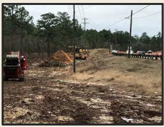
The Clemson Road Widening project began in February and clearing and grubbing operations are underway.
