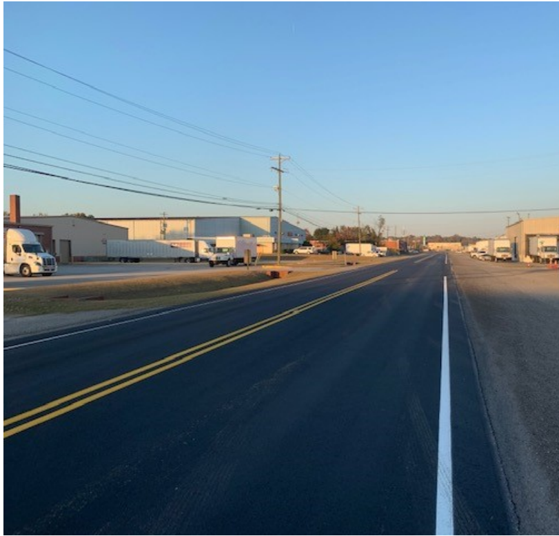
Rosewood Drive Resurfacing (RESURFACING PACKAGE "R")
